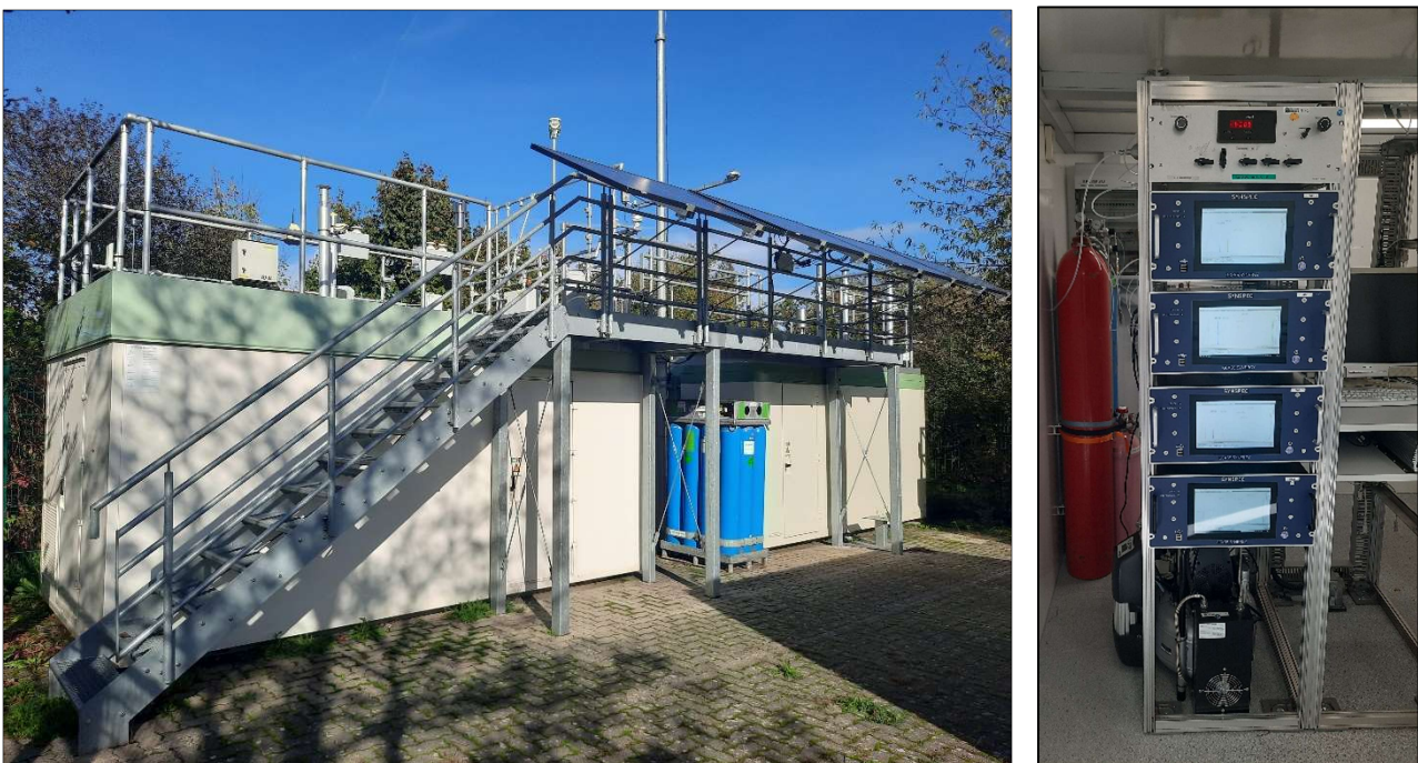
Fig. 4.1: Measuring station at the LUBW test site
