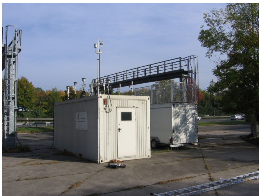
Figure 24: Field test site Bornheim, motorway parking lot
